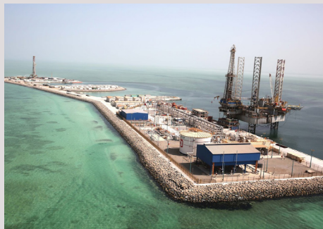
The Hail Site Terminal - Abu Dhabi Oil Co Ltd's latest site. The crude oil produced is sent to Mubalas Island through a submarine pipeline for final processing prior to product shipping. © Abu Dhabi Oil Co Ltd
