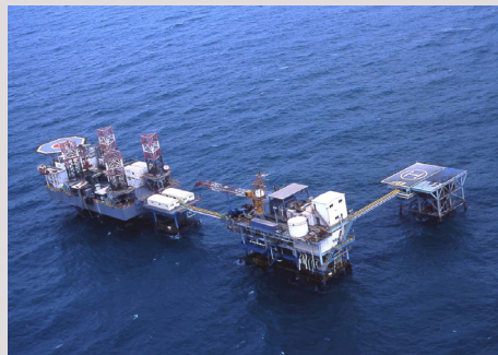
Mubalas Central Facilities Platform (CFP). Crude Oil produced from each production well is sent to Mubalas Island through a submarine pipeline via this CFP. © Abu Dhabi Oil Co Ltd
